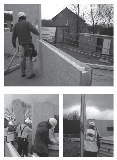
Fig. 1.18. SIPs during construction.
