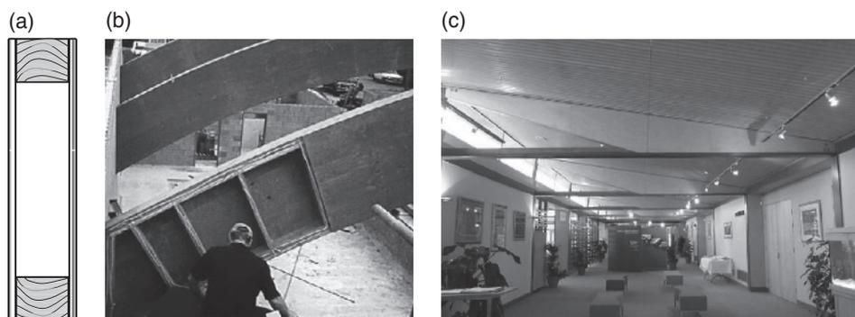
**Fig. 1.17.** Box beam: (a) cross-section, (b) curved ply-box beam during construction (photo courtesy of Peter Yttrup and Fred Bosveld), and (c) tapered ply-box beam (photo courtesy of Catriona McLeod and Port of Brisbane Corporation, Australia).
