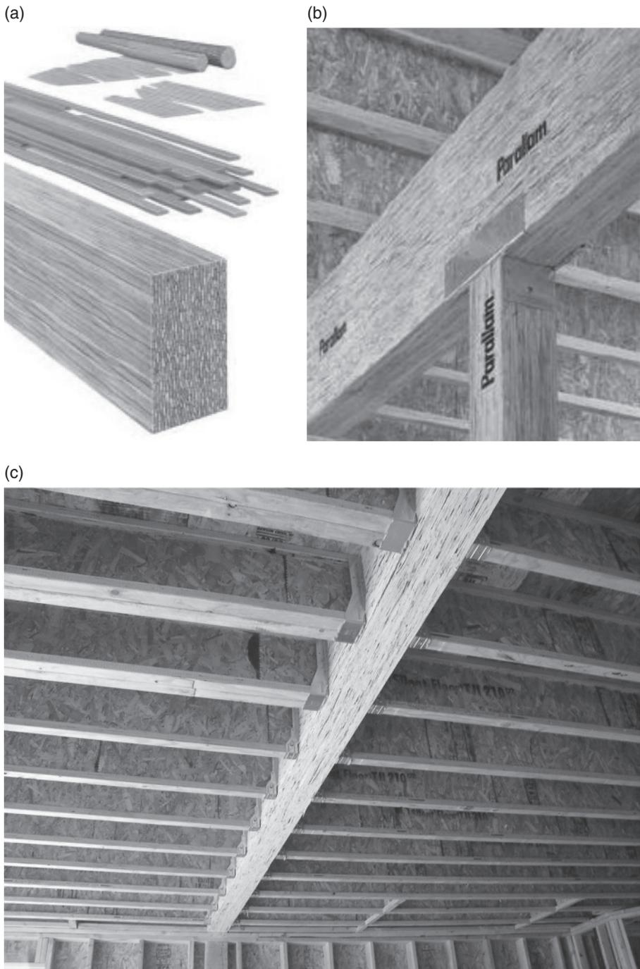
**Fig. 1.14.** Parallam (PSL) – manufacturing process and in construction; photos (a) and (b) courtesy of Weyerhaeuser.
