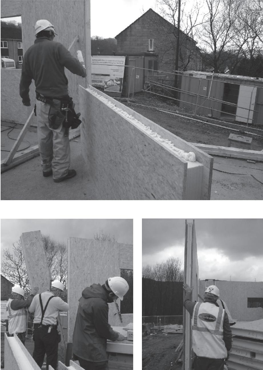
**Fig. 1.18.** SIPs during construction.
