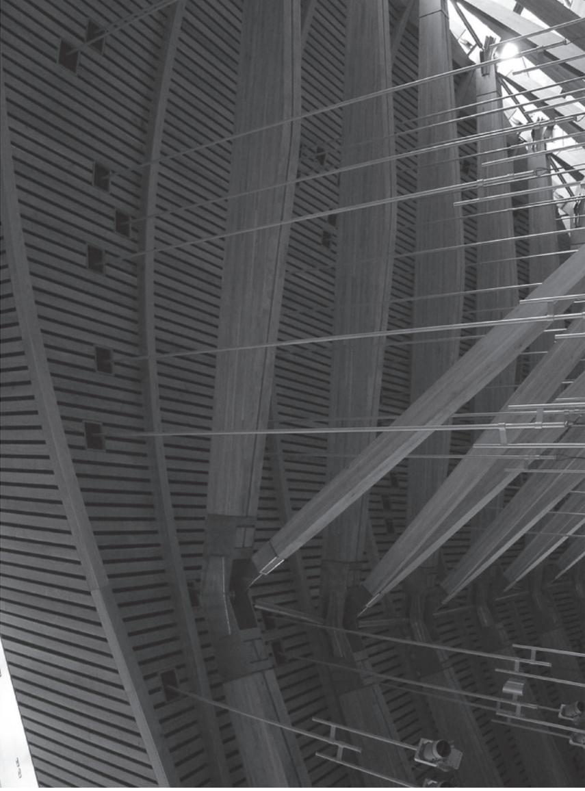
**Fig. 1.8.** Glued-laminated structures. (Part (b) photo courtesy of APA, The Engineered Wood Association. (c) photo courtesy of Axis Timber Limited, a member of the Glued Laminated Timber Association, UK.)
