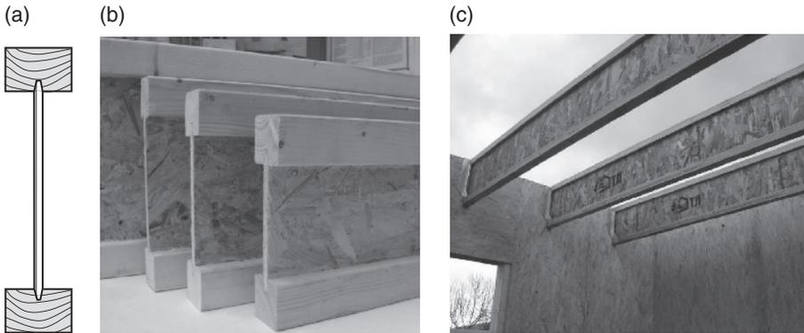
**Fig. 1.16.** Typical I-joists and their application.
