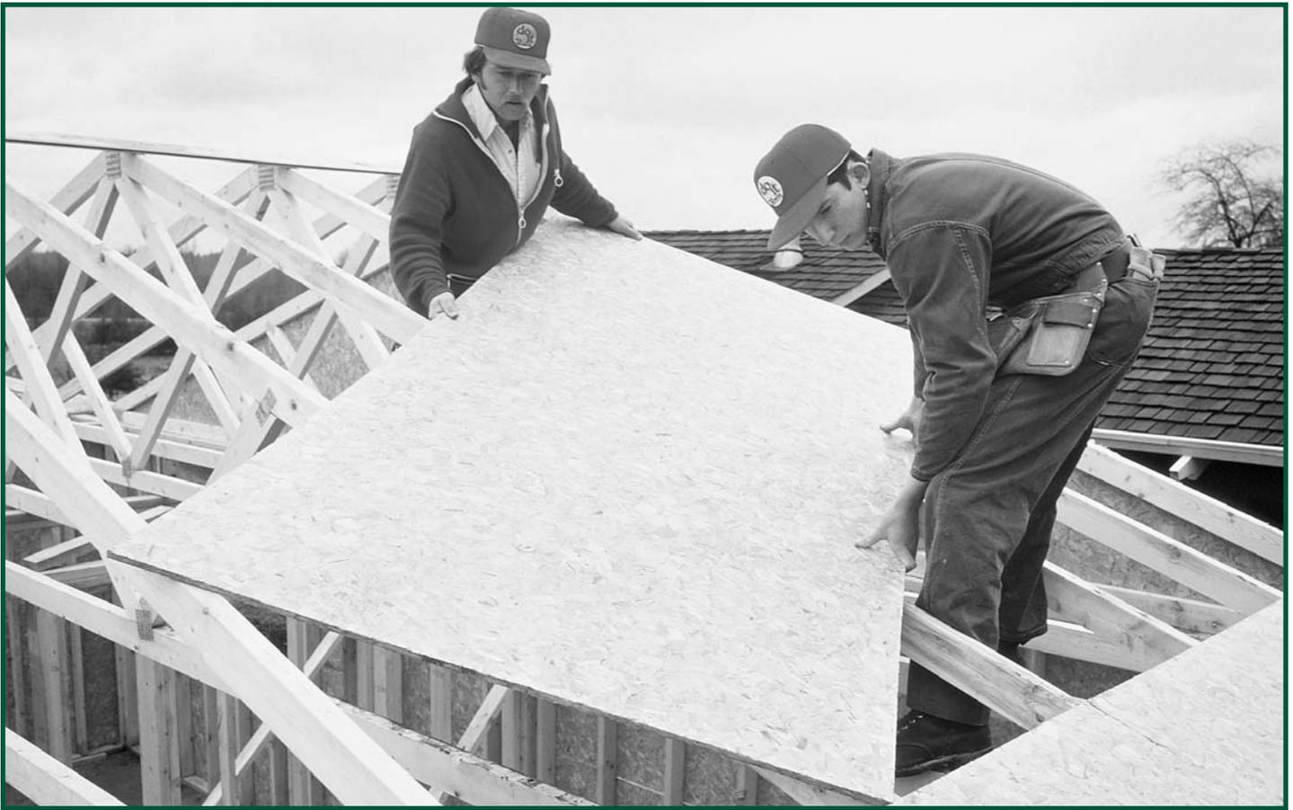
The panels should be installed textured side up with their long direction across the rafters or truss chords. Long panel edges should be supported or joined with edge clips where required. A 1/8" gap should be left at the panel edges and ends to allow for movement due to changes in humidity. Panels should be staggered at least two supports and end joints must lie over supports.
