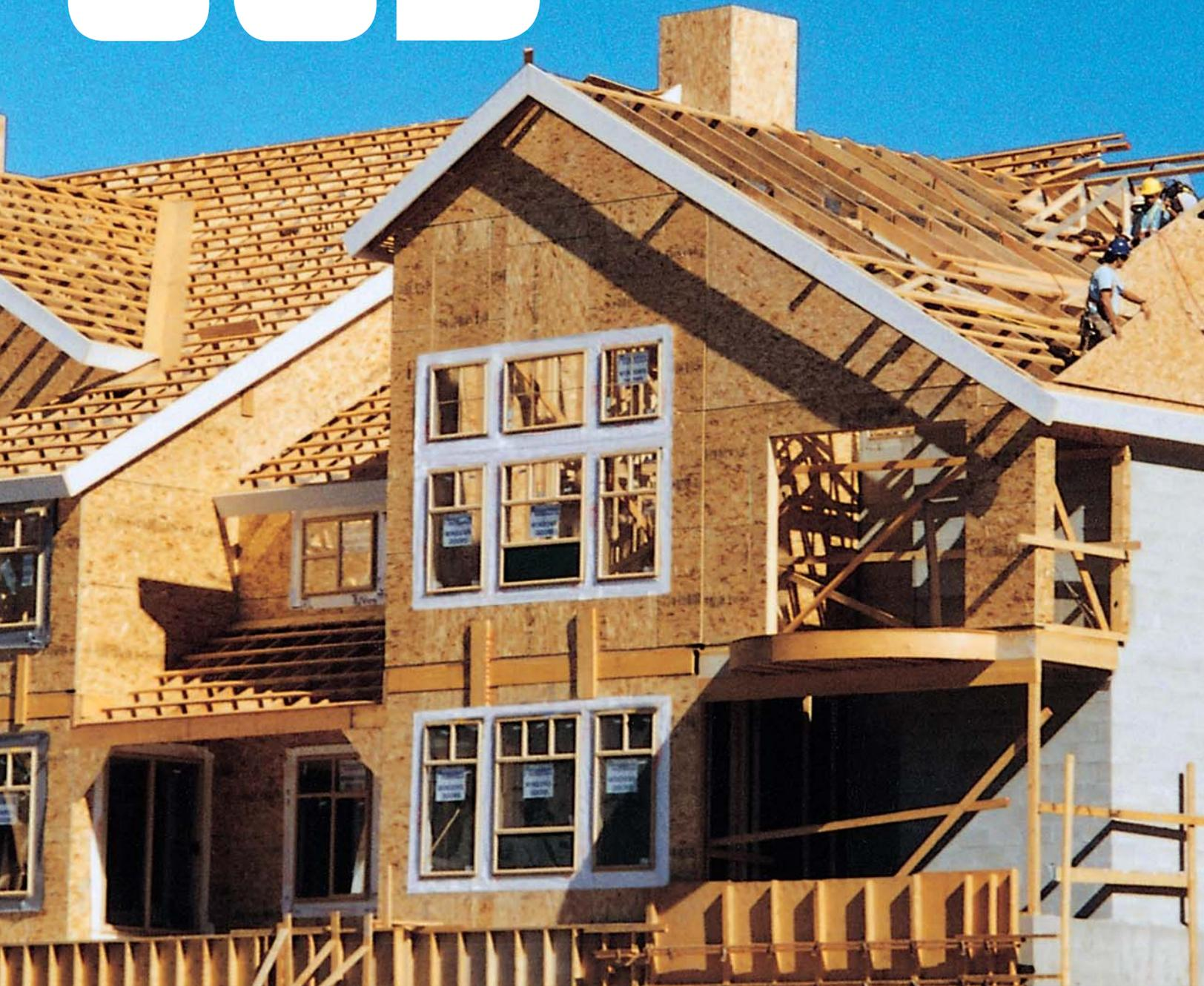
**OSB IN WOOD FRAME CONSTRUCTION**
